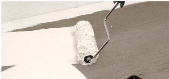
INTERIOR concrete slabs prior to flooring.
