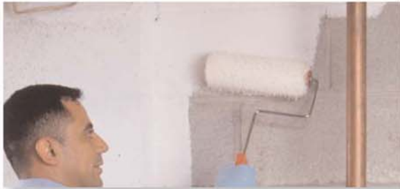
INTERIOR concrete and masonry basement walls.
