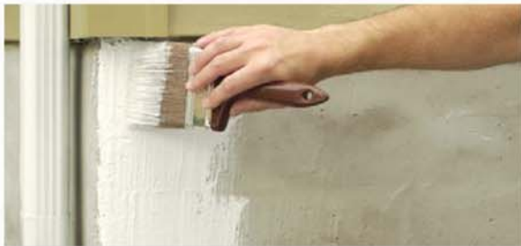
EXTERIOR above and below grade concrete, stucco and masonry foundations.
