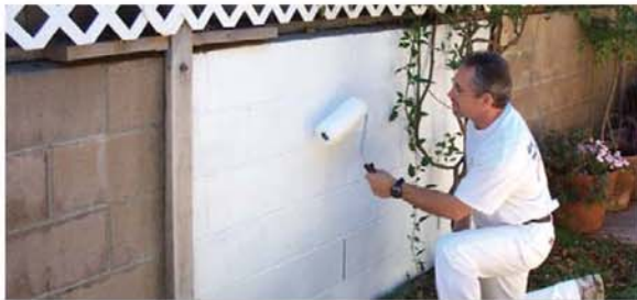
EXTERIOR retaining walls.
